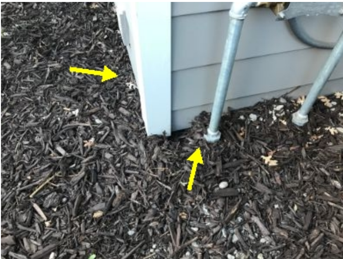
Keep bark away from composite siding to minimize moisture damage and pest issues.
