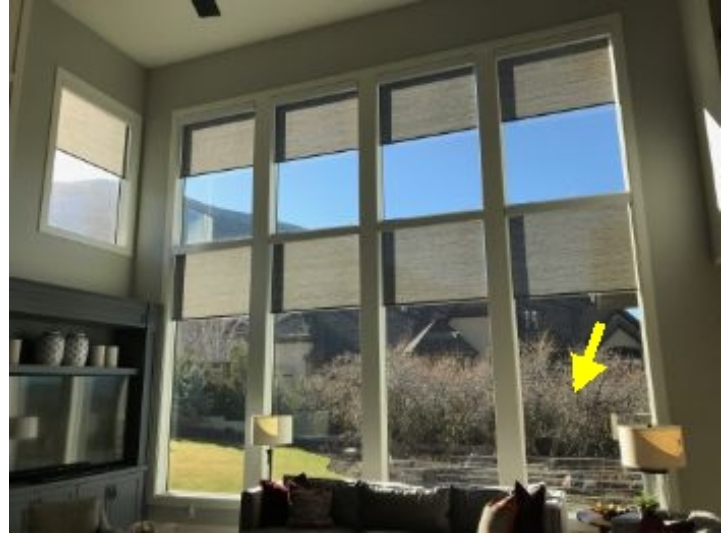
Numerous areas where glass is etched/scratched on outside of large south windows.
